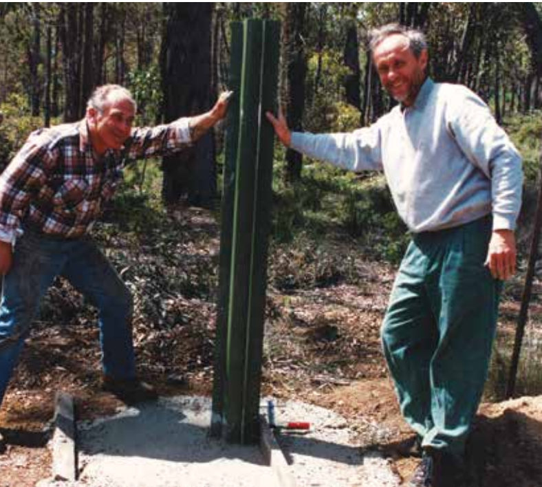
Hands on during the fence construction at Karakamia
