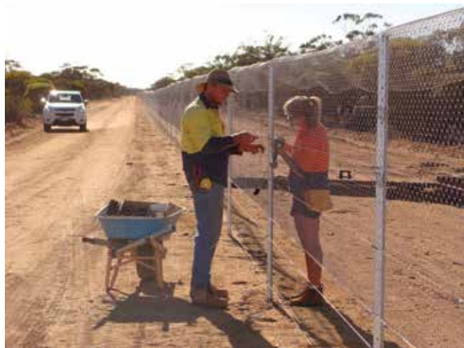
Insulators being fitted on the electric wires M McFall
