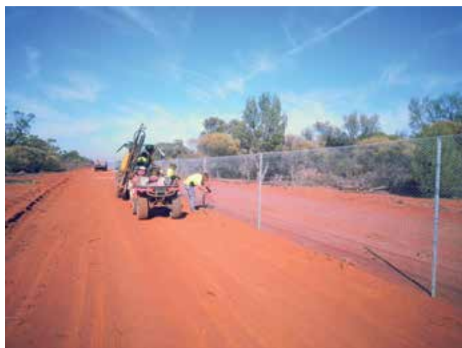
Installation of skirting M McFall
